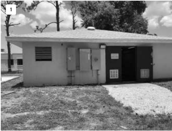
Project: SA-23-2007-REP (DKI) Date: 6/6/2023, 1:43pm Creator: Robert Patton Tags: utility room
