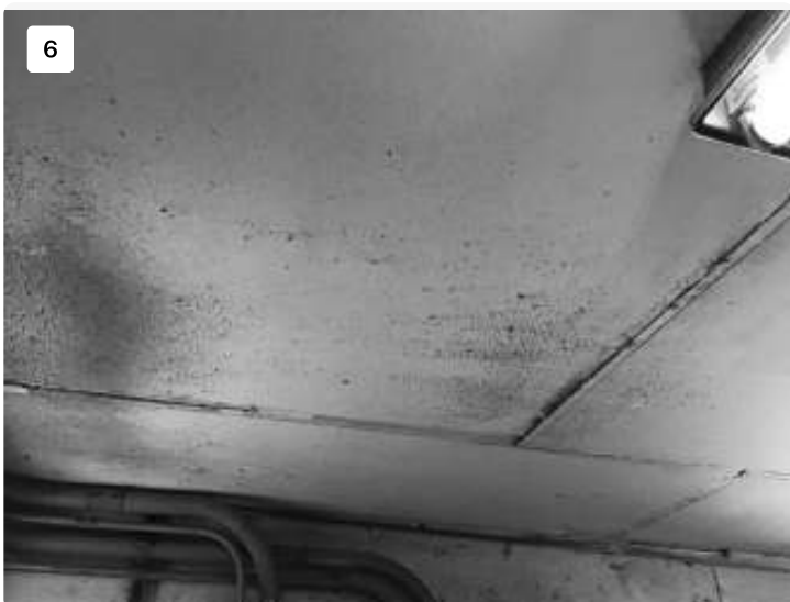
Project: SA-23-2007-REP (DKI) Date: 6/6/2023, 1:59pm Creator: Robert Patton Tags: utility room
